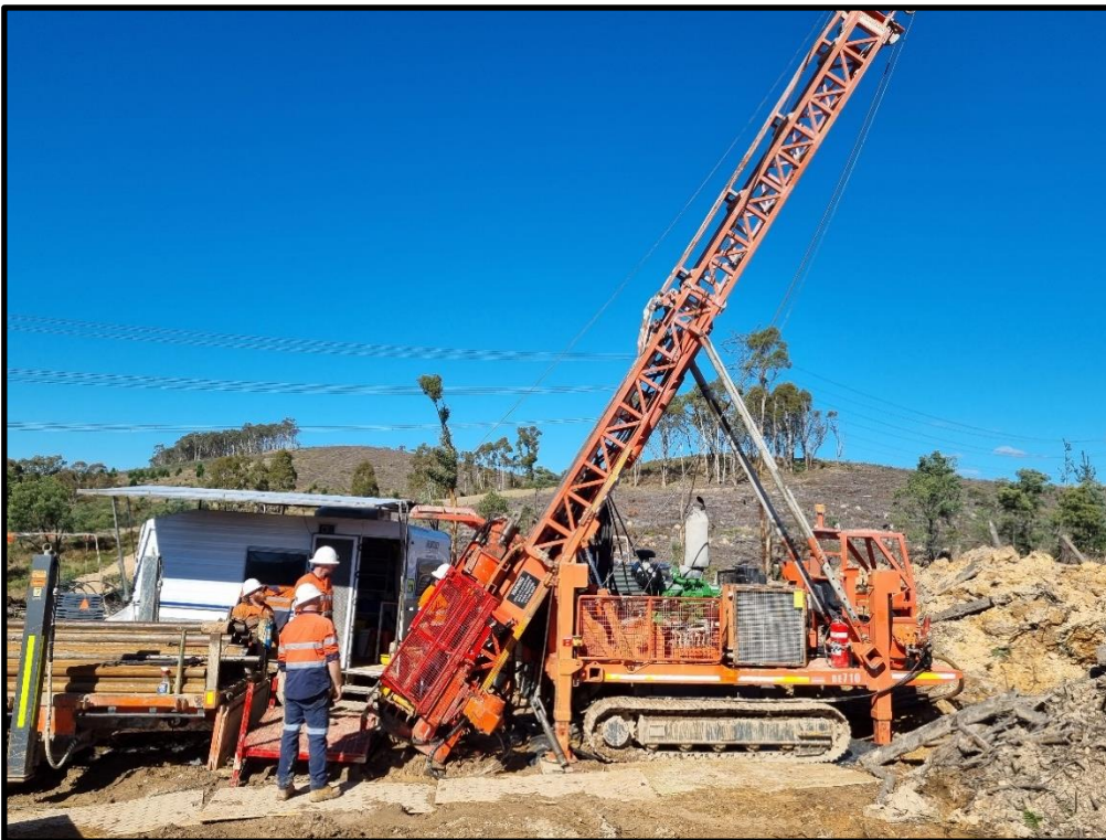
Figure 2- Diamond drill rig set up on first hole
